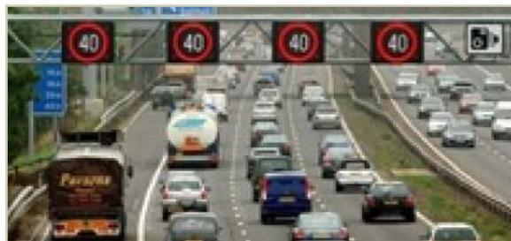
With spacing between emergency refuge areas extended from 800m on the M42 pilot scheme to a new standard of up to 2500m, cars could be limping along for up to 1.5 miles in fast traffic.
